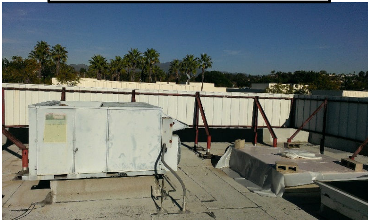
EXISTING – PACKED RTU
