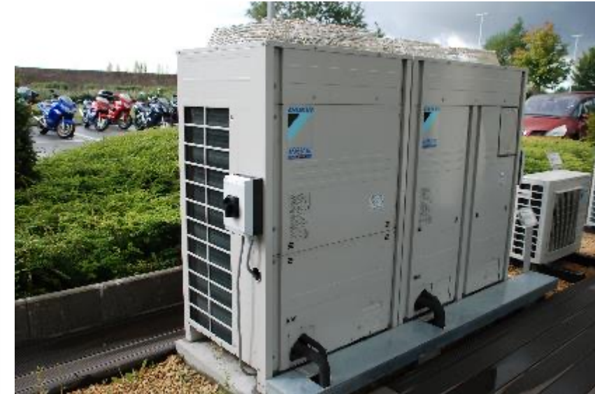
VRF Using R-32 Refrigerant
