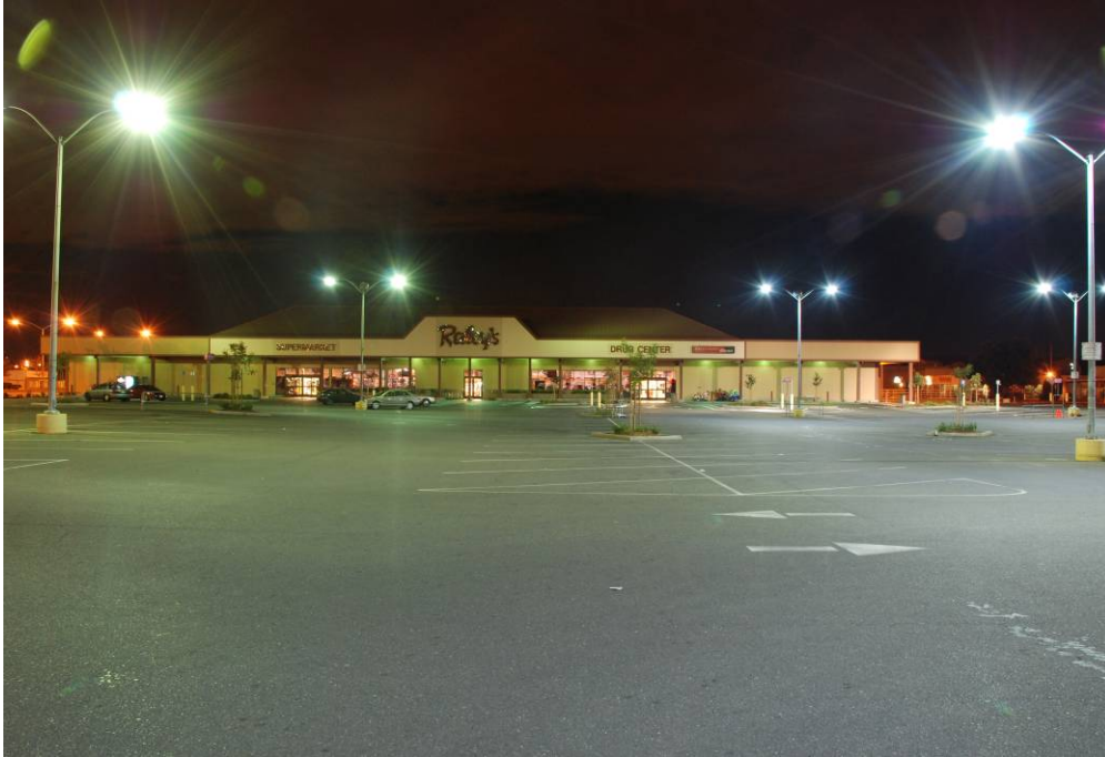
Figure 9: Comparison of MH Luminaires (Left) and LED Luminaires on High Power (Right)
