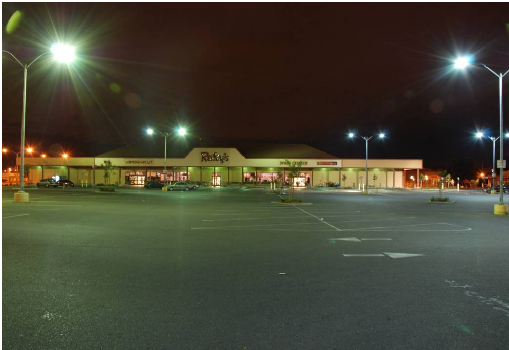
Figure 10: Comparison of MH Luminaires (Left) and LED Luminaires on Low Power (Right)
