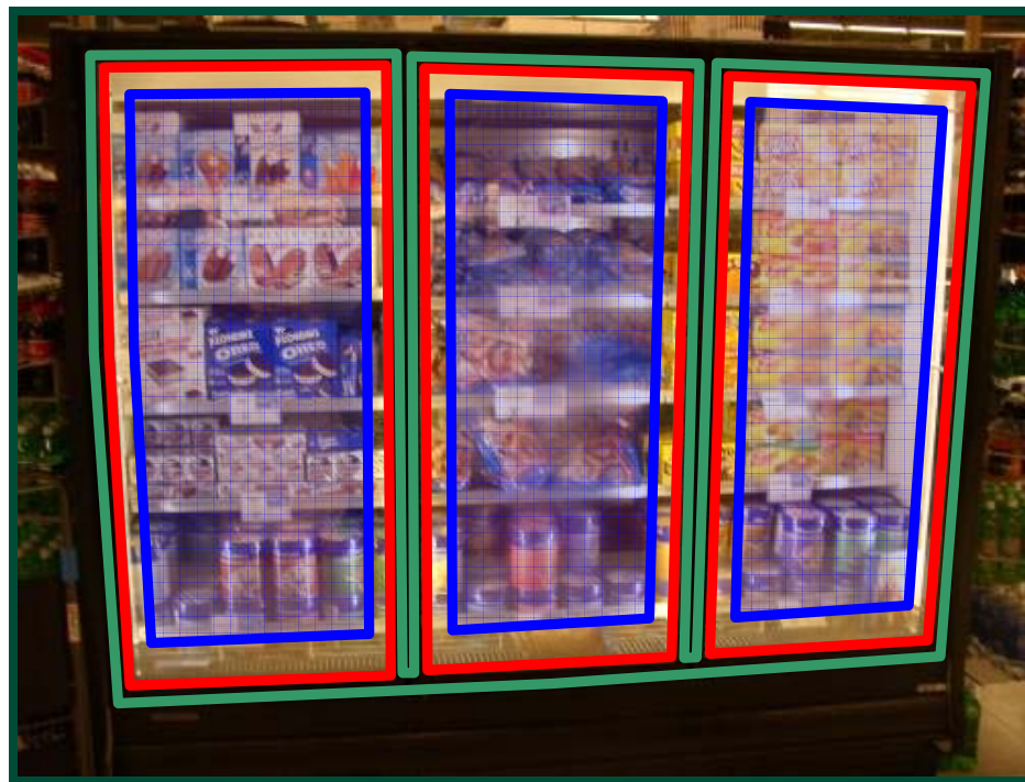
FIGURE 3. TYPICAL ANTI-SWEAT HEATERS LOCATION FOR LOW-TEMPERATURE REACH-IN DISPLAY CASES
