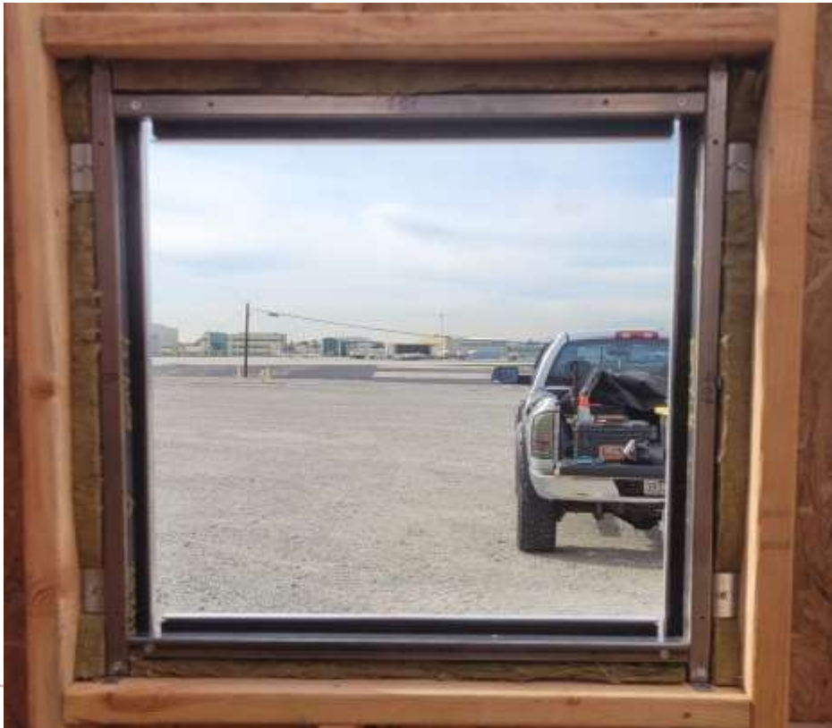
Interior View – Ready for Glazing
