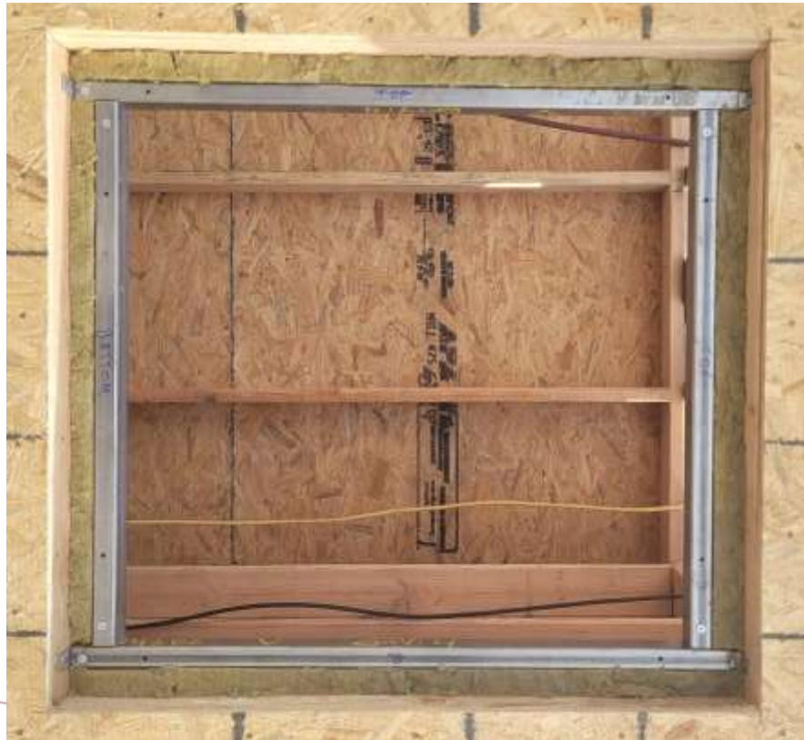
Mineral Wool – Thermal Barrier
