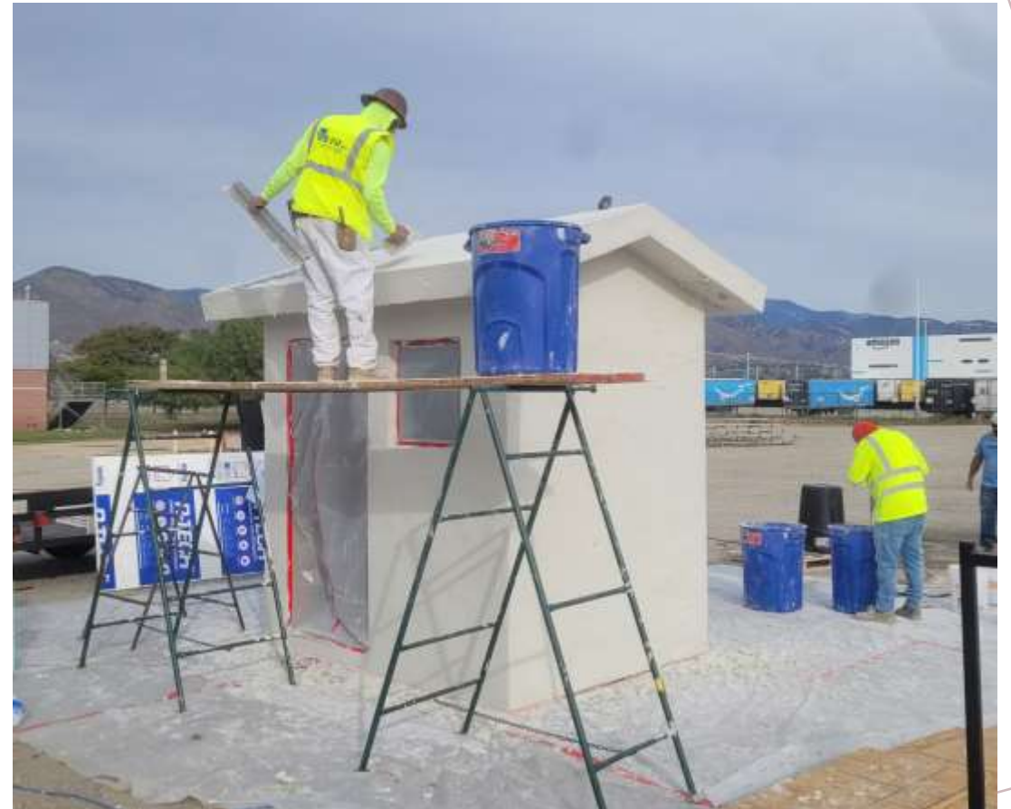
U-Stucco being installed.
