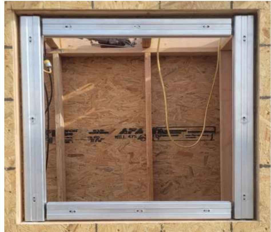
Gypsum Filled Aluminum Caps
