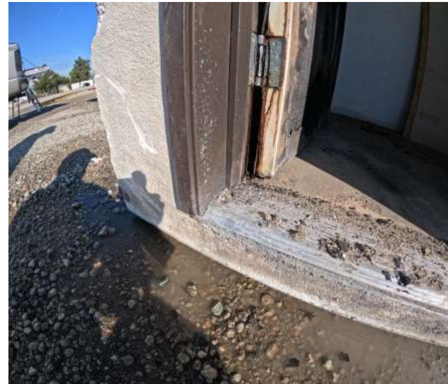
Aluminum threshold survived (melts at 1,221 degrees F)
