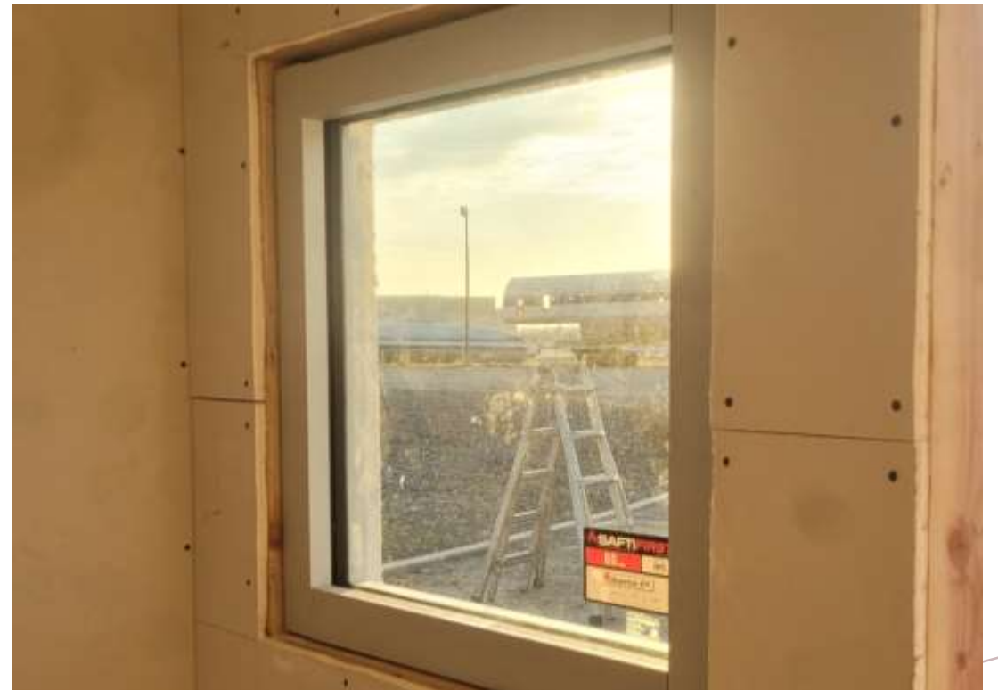
Drywall & Taped for Air Seal
