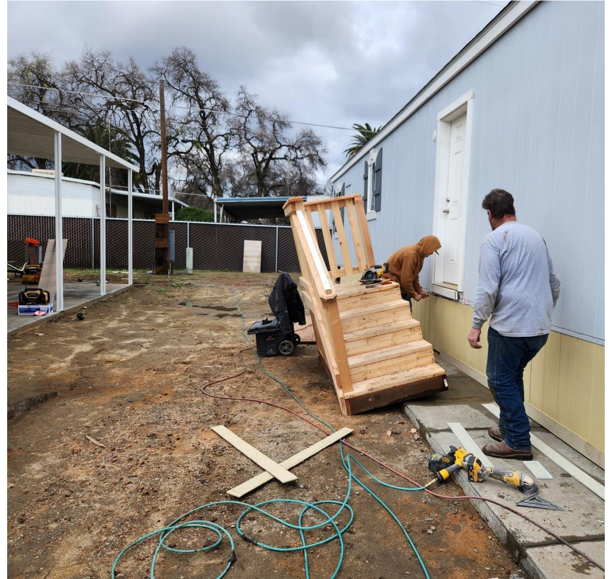
Set up at Visalia manufactured home park. EPRI. 2022.
