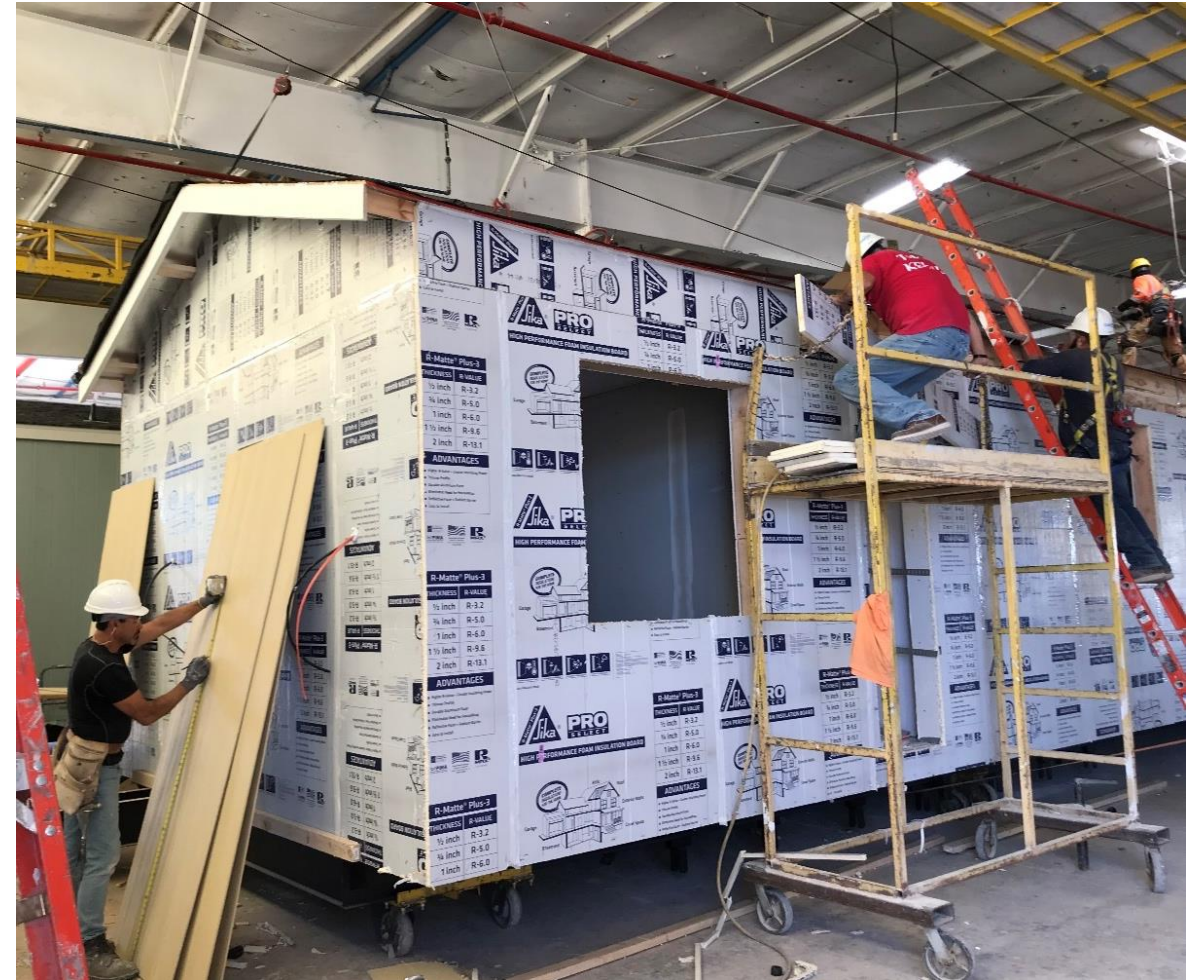
Rigid foam board installation at plant. EPRI. 2022.
