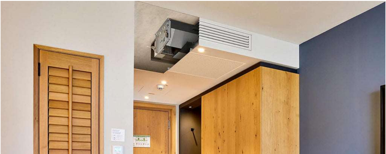
Figure 14: Mechanical Indoor Unit Installation
