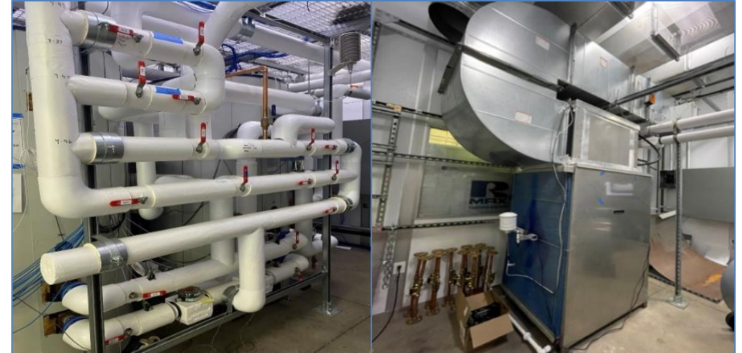
Heat Pump Water Heater System Testing
