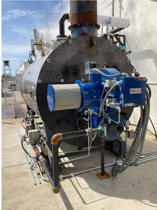
Figure 1. Industry Standard ULNB – Mesh Burner
