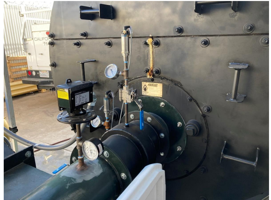
Figure 2. Rogue NZN Burner with ClearSign Core Technology
