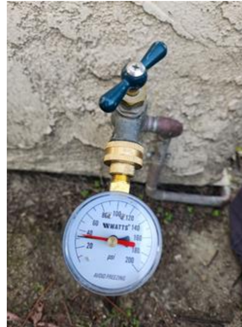
(L) Low water pressure DHW system #1
