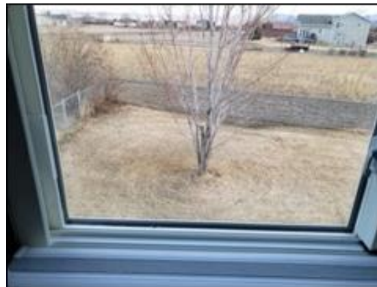
Window replaced with Thin-triple
