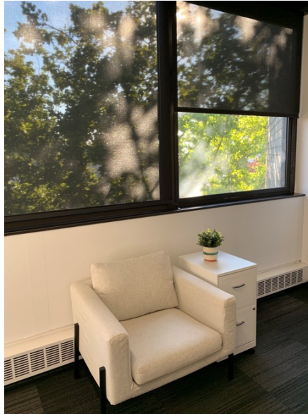
After: Integrated Solar Shades
