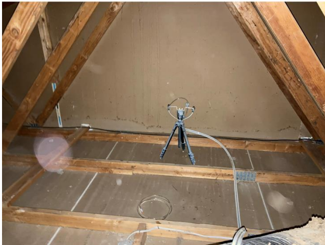
1. Seal attic/crawl space
