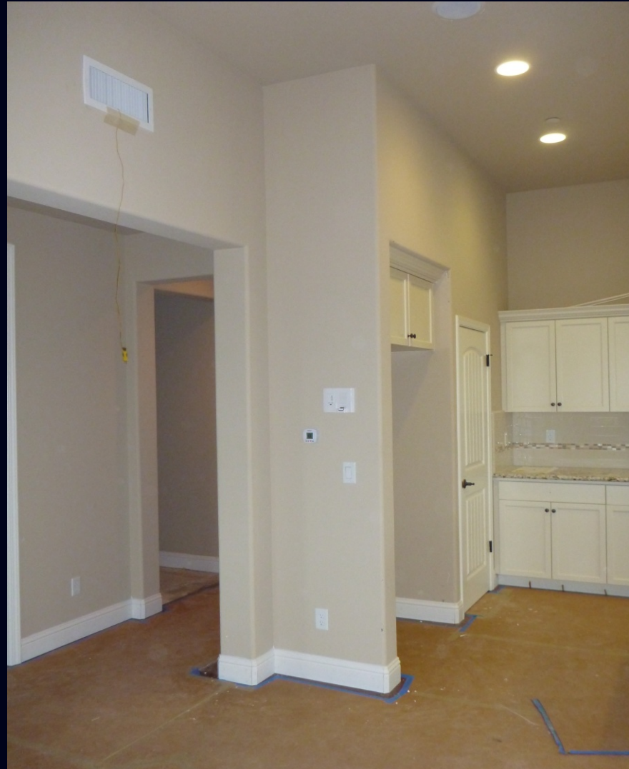
Source: PG&E ET Project field observation
