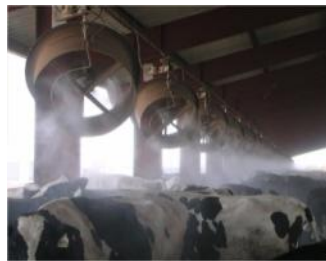
FIGURE 12. HIGH PRESSURE MISTING SYSTEMS
