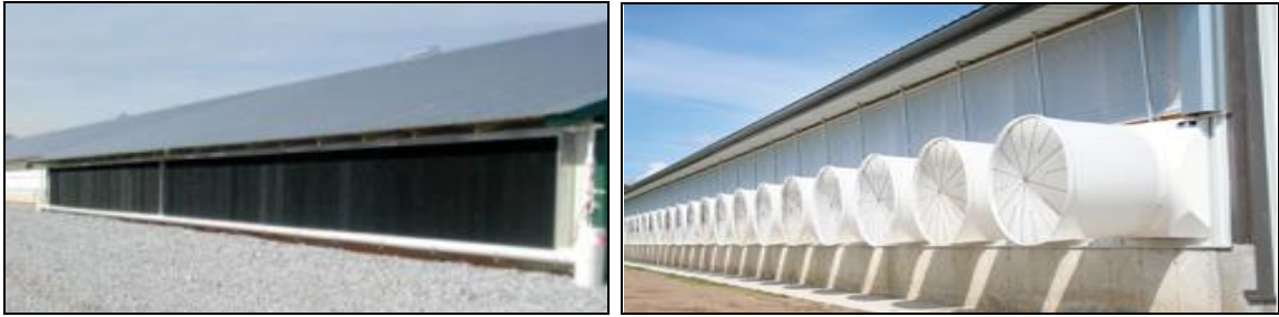
FIGURE 14. PICTURES SHOWING INSTALLATION OF AQUACOO ® EVAPORATIVE COOLING SYSTEMS
