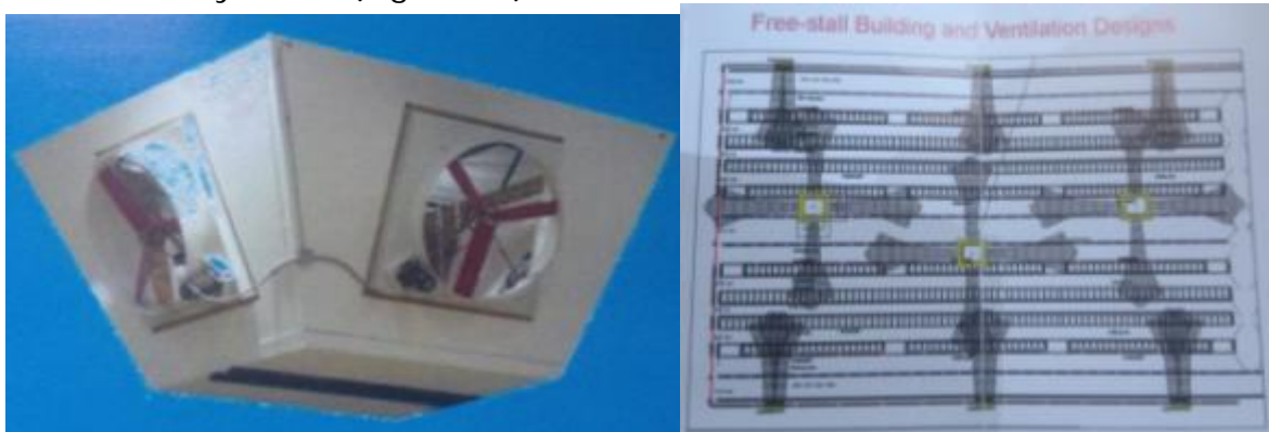
FIGURE 16. PICTURE OF FANS USED FOR TURBULENCE VENTILATION
