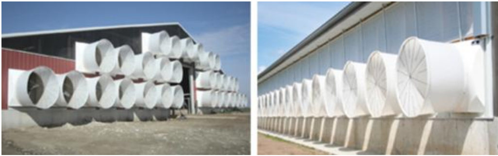
FIGURE 5 .TUNNEL VENTILATED BARN (LEFT) AND CROSS-VENTILATED BARN (RIGHT)
