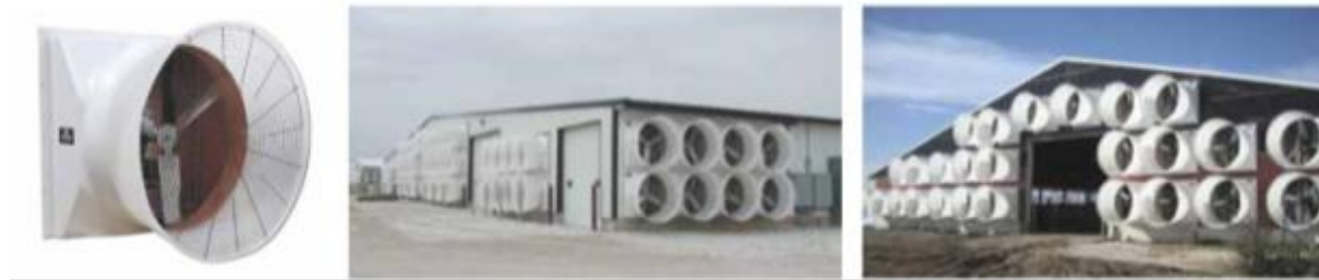
FIGURE 10. EXHAUST FANS USED IN CROSS AND TUNNEL VENTILATED BARNs (PHOTO COURTESY: SCHAEFER FANS)
