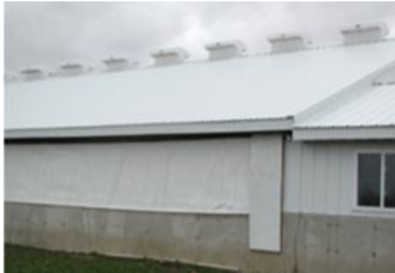
FIGURE 17. PICTURE SHOWING VENTILATION ROOFS
