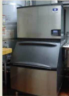
ENERGY STAR replacement ice machine.
