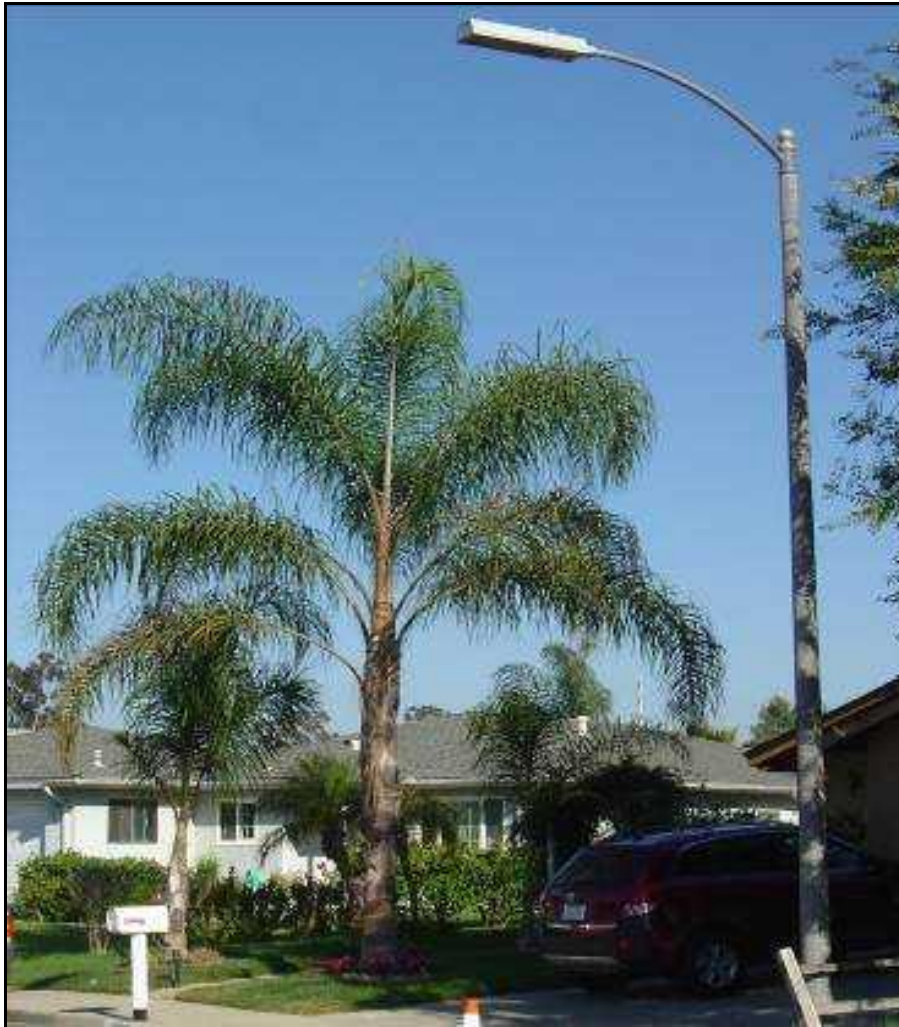
Figure 1: Existing LPS luminaire on Lindsley Park Drive
