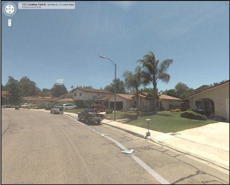
Figure 3: Induction luminaire at Lindsley Park Drive
