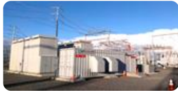
Distribution Level Energy Storage
