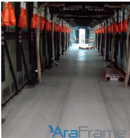
Hot aisle - Cooling coils in top of hot aisle
