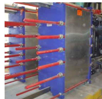
Segregate cooling tower water from data center cooling coils
