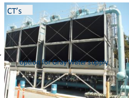
Segregate cooling tower water from data center cooling coils
