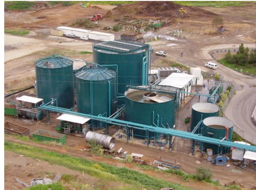
Today's Anaerobic Treatment
