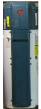
Heat Pump Water Heater
